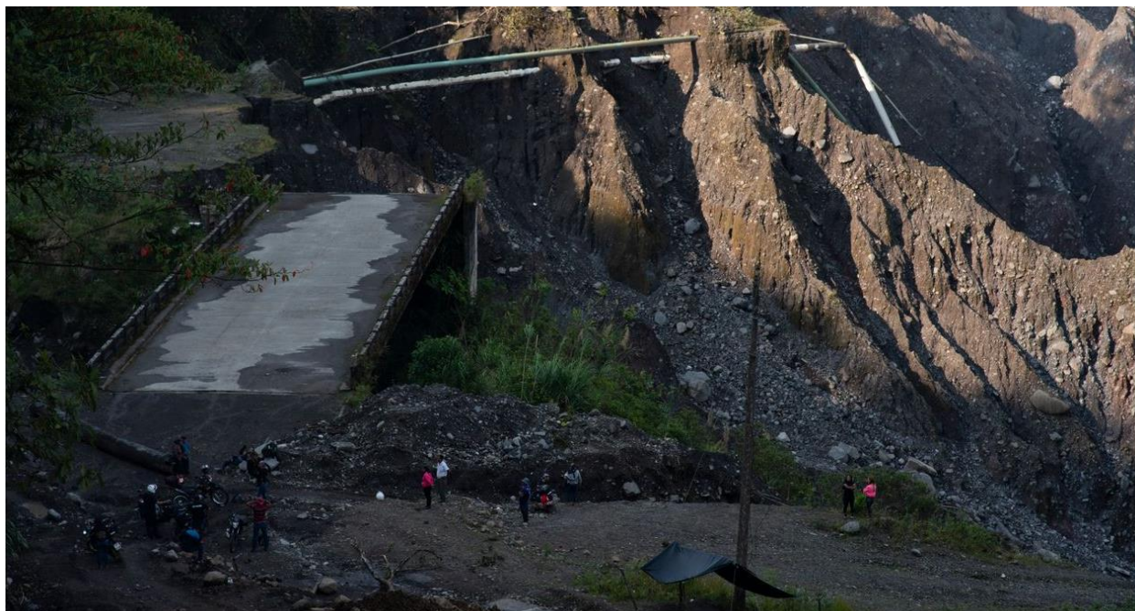
Erosion along Ecuador’s Coca River, which some geologists blame on the Coca Codo Sinclair plant, has destroyed stretches of a highway, an oil pipeline and part of a nearby town.
